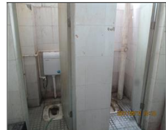
Photo of the sanitary facilities Toilet.JPG
