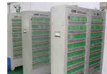
Battery Capacity Detection Cabinet
